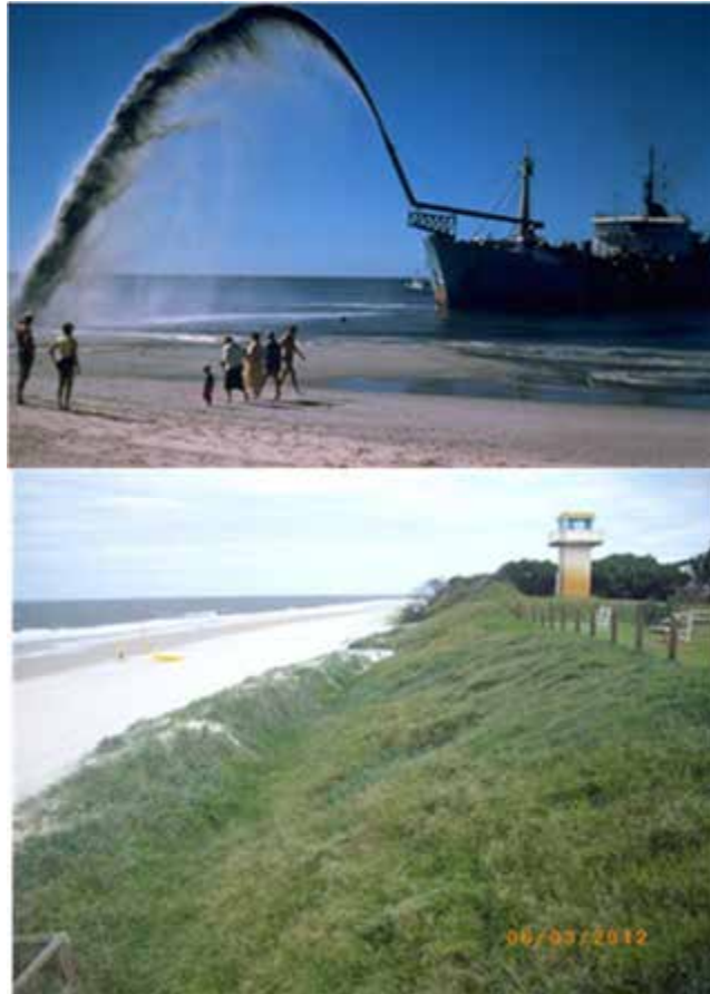
Figure 5 Beach nourishment in Queensland. Top: “rainbowing” sand from a dredge at Woorim, Bribie Island, circa 1988.; Bottom: Stabilised beach at Woorim in 2012. Source: Beach Protection Authority and GHD Pty Ltd.
