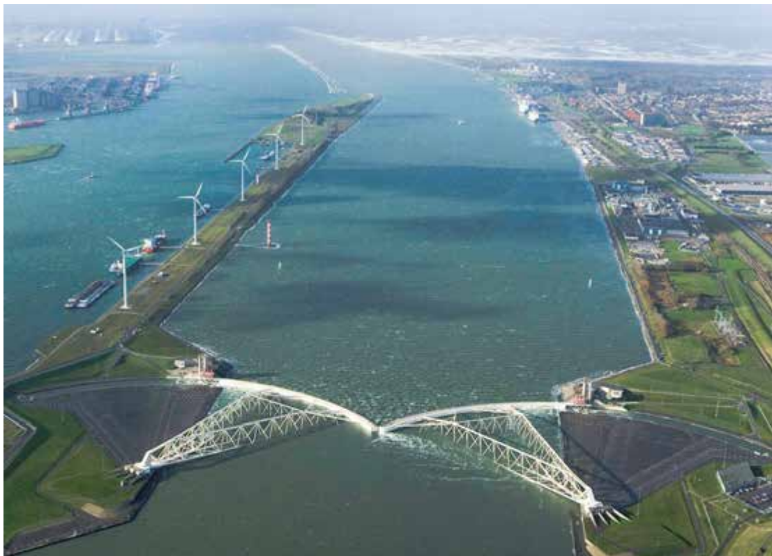
Figure 33 Storm surge barrier at the Port of Rotterdam, The Netherlands Source: Netherland Ministry of Water and Public Works www.rijkwaterstaat.nl
