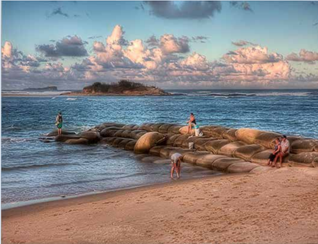
Figure 24 One of the four geotextile groynes at the Maroochy river mouth, on the Sunshine Coast.
